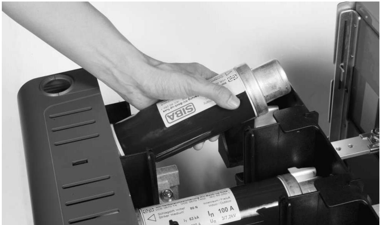
Fig. 4.2 Replacing the fuse
