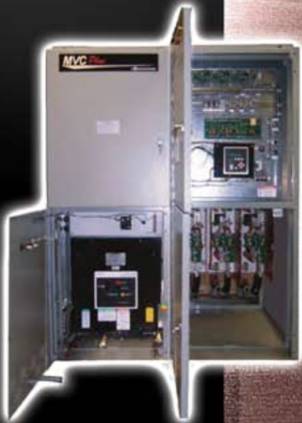
4160V, 1000A Soft Starter with Synchronous Controller for 10,000 HP gas compressor.
